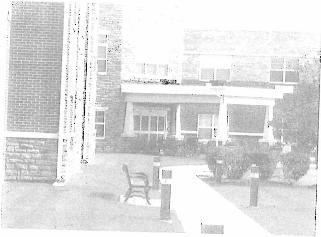
Main Entrance to Nursing Home
