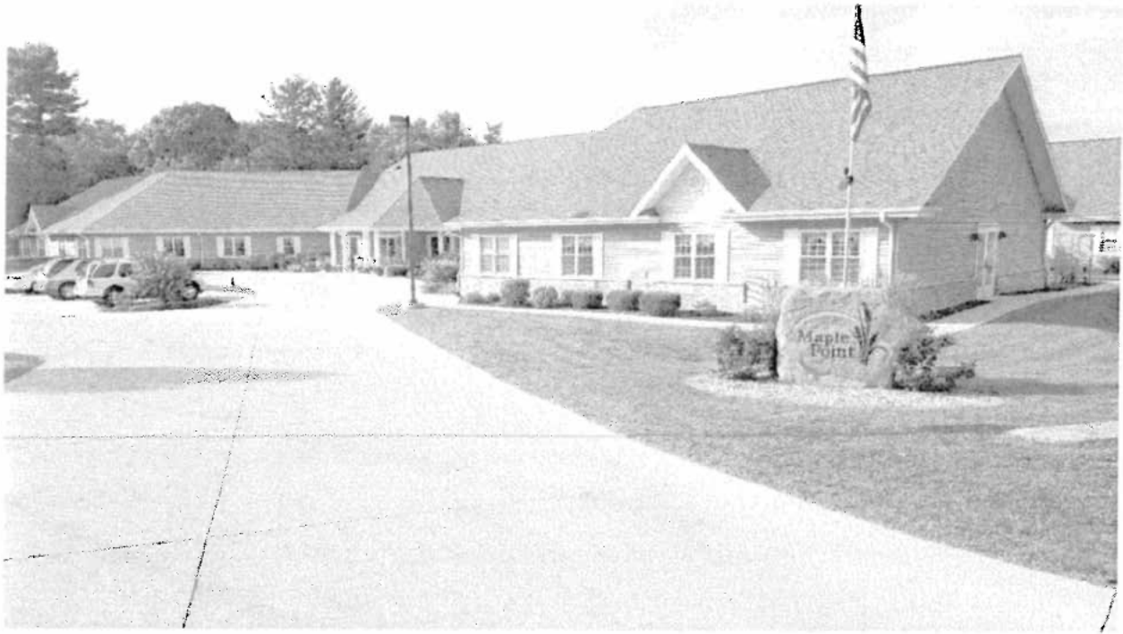
Front entrance from driveway
